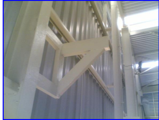
Pipe Support install work
