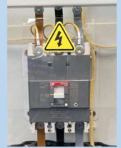
8 - ABB Circuit Breaker
