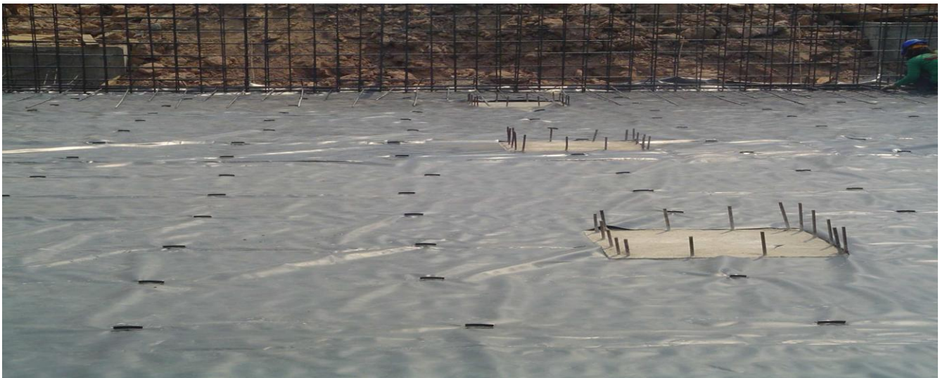
LDPE Sheet Sub-layer installed before Concrete pouring
