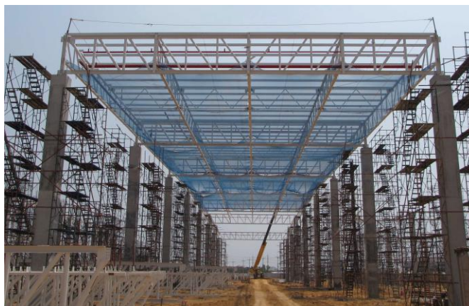
Installed Safety Nets
